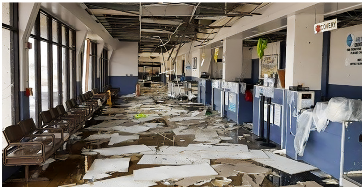
Destruction inside the Francisco C. Ada Saipan International Airport after Typhoon Yutu passed over the island. Photo by FEMA, 2018, courtesy of CNMI Office of Planning and Development.
